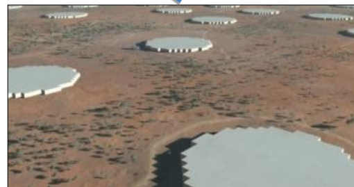
SKA2_AA 250 x Mid Frequency Aperture Array Stations
